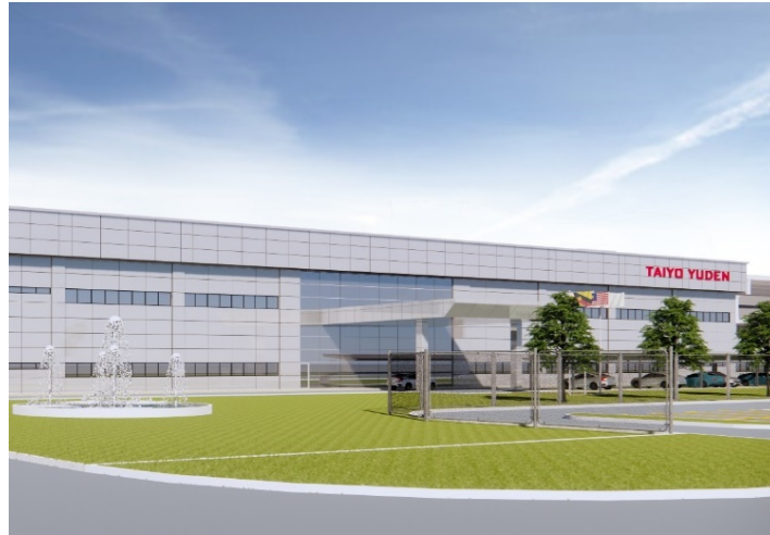
Conceptional drawing of the new plant at TAIYO YUDEN (SARAWAK) on completion
