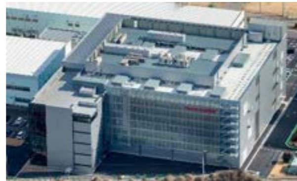
Exterior of the materials building at Yawatabara Plant (Takasaki City, Gunma Prefecture)
